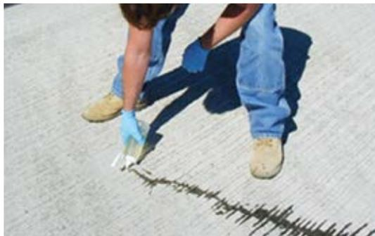
*Flood surface with properly mixed epoxy*
