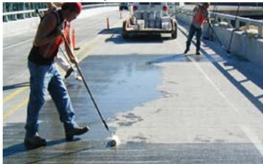
*Remove excess epoxy and immediately apply fine sand into the wet epoxy*
